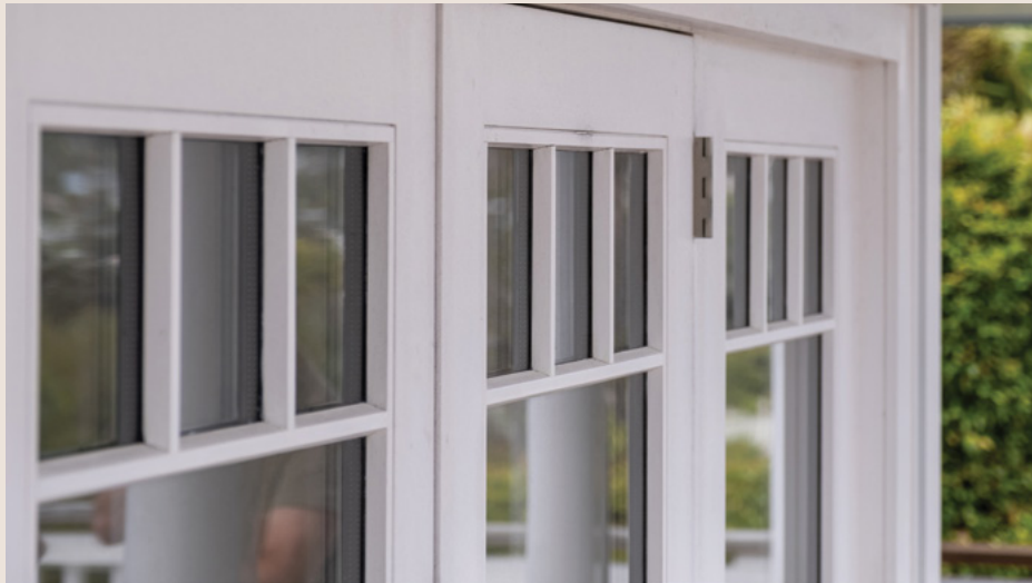
○ Vulcan window joinery Whangaparoa, New Zealand. Installed 2010.
