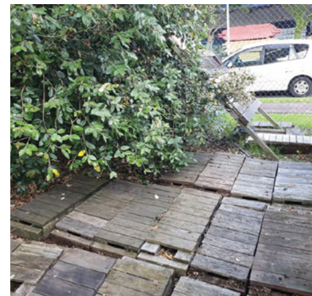
○ Decking test panels, Mangere.
