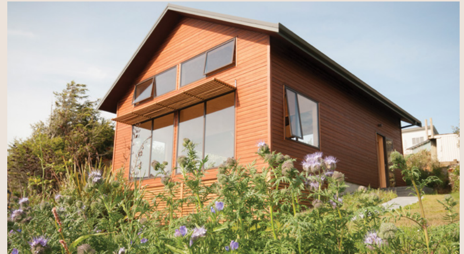
○ Vulcan Cladding (Vertical Grain) – Raglan, New Zealand. Installed 2013.
